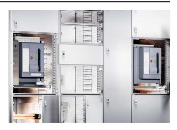
In addition to the ACB, control and measurement equipment with a maximum heat loss of 50 W may be installed in the circuit-breaker section.
